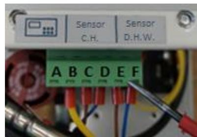
PIN 1 – black, steering; PIN 2 – blue, neutral; PIN 3 – brown, line; Connection of the D.H.W. sensor – PIN E I F
